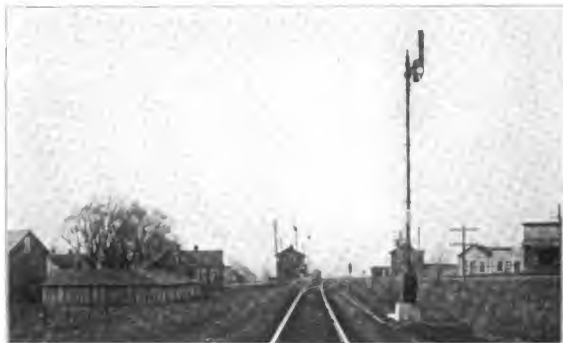
WEST BRANCH FROM THE SOUTH, SHOWING BLOCK SYSTEM ON THE C. R. I. & P. R. R.
